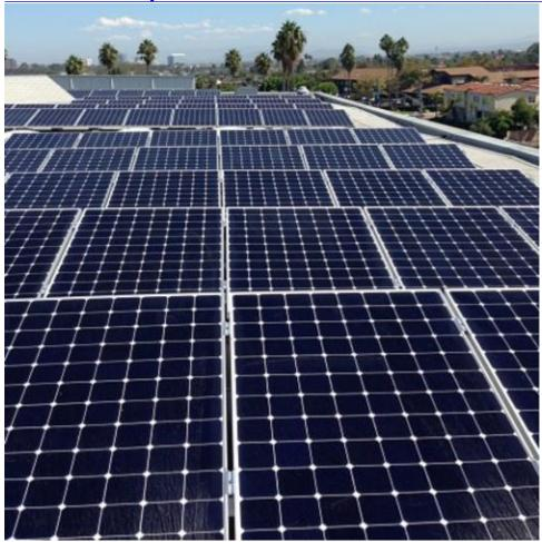
Installed for less than \$144,000 in late 2014, 152 solar panels and three inverters provide the vast majority of electricity needs for San Diego's Our Mother of Confidence Parish. The estimated pay-back period for initial costs is five years. (Courtesy of Our Mother of Confidence Parish)
