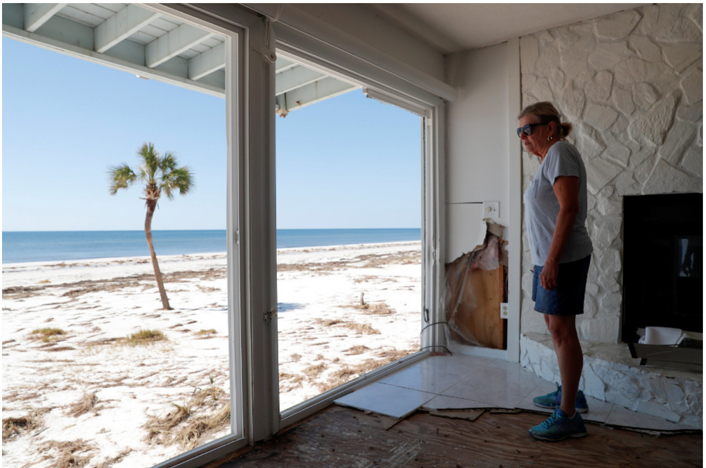
Katherine Shimonis, 69, stands in her damaged living room Oct. 18 in Port St. Joe, Florida, in the aftermath of Hurricane Michael. (CNS/Reuters/Terray Sylvester)
