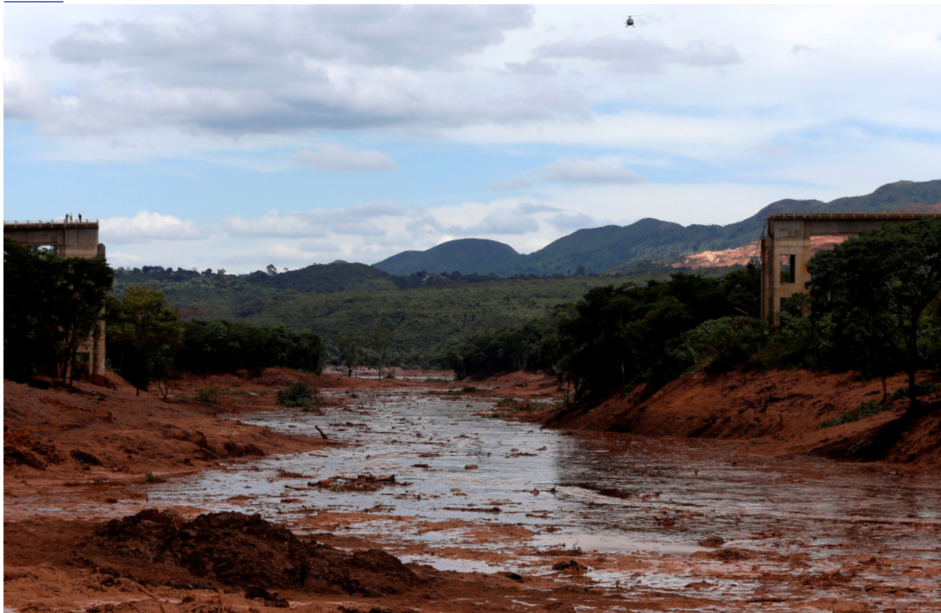
A view of the aftermath from a failed iron ore tailings dam in Brumadinho, Brazil Jan. 27, 2019. (CNS/ Reuters/ Adriano Machado)
