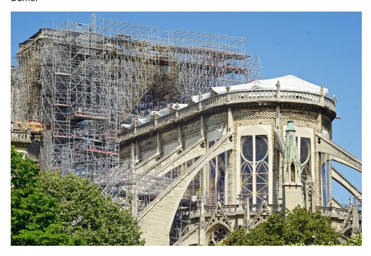
A view of the eastern end of Notre Dame Cathedral on June 15, 2019, showing the choir area where the glass has been removed from windows now stabilized by wooden supports. The white plastic sheeting on top protects replaces the burnedaway roof. The scaffolding above the cathedral was put up during the renovation
