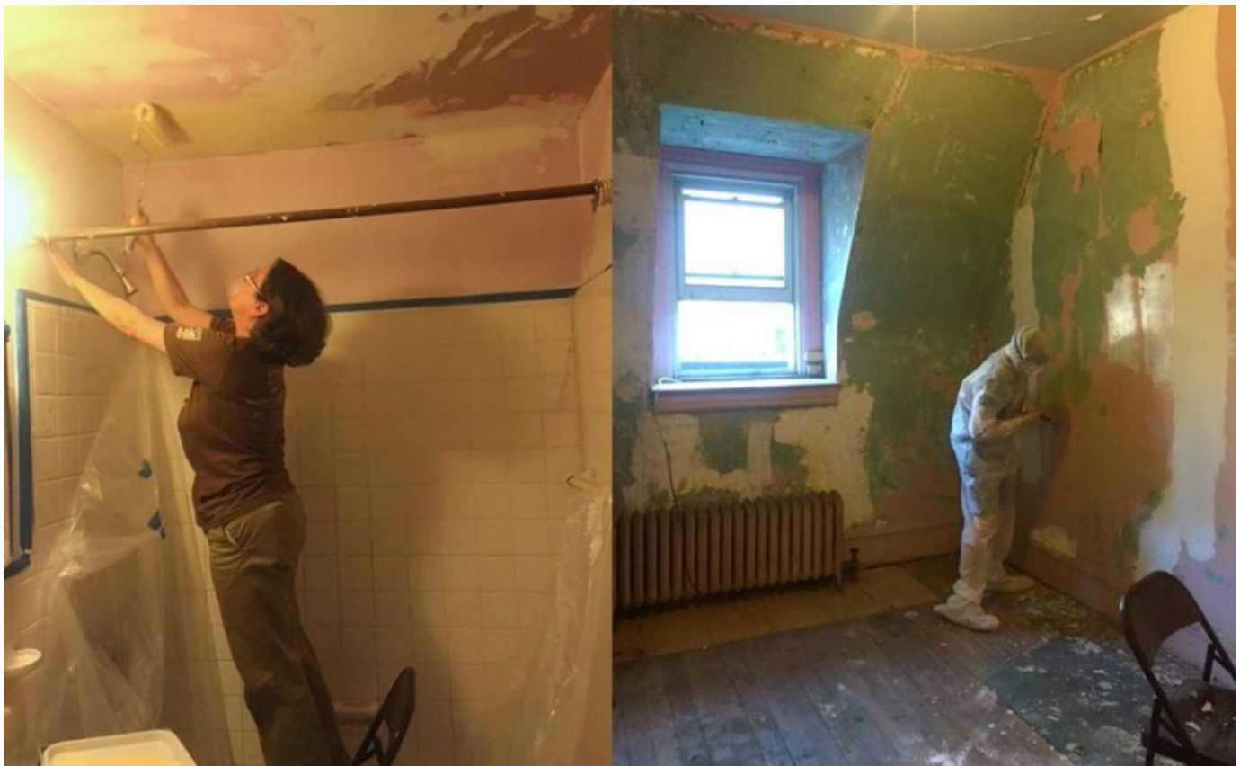
Left: St. Joseph Sr. Susan Wilcox paints the ceiling in one of the convent's bathrooms; right: Volunteer Sarah Brook had to wear protective clothing to restore one of the convent's bedroom. (Courtesy of Benincasa Community)
