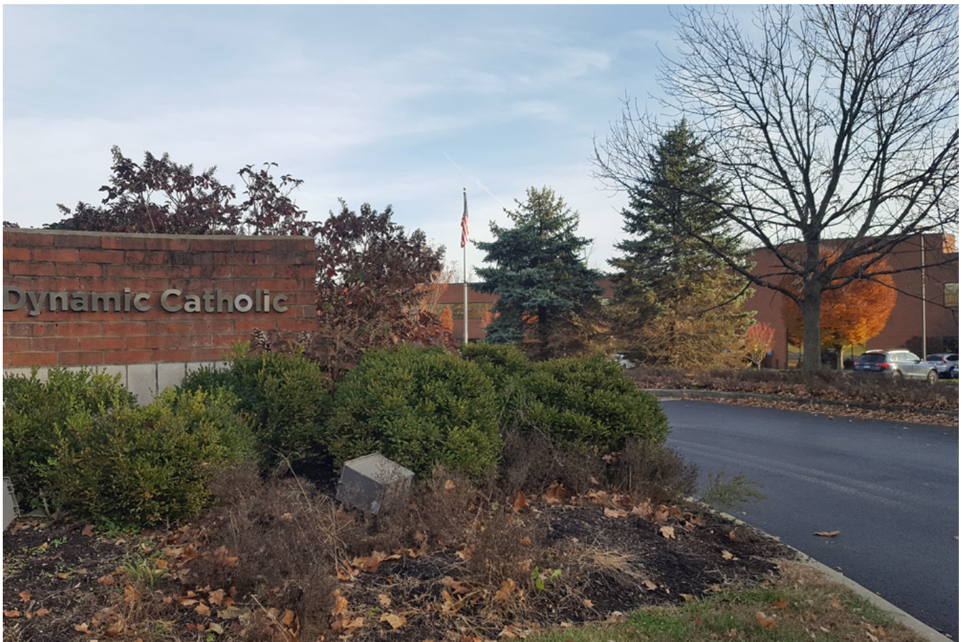
Exterior of the Dynamic Catholic Institute building in Erlanger, Kentucky (NCR photo/Heidi Schlumpf)
