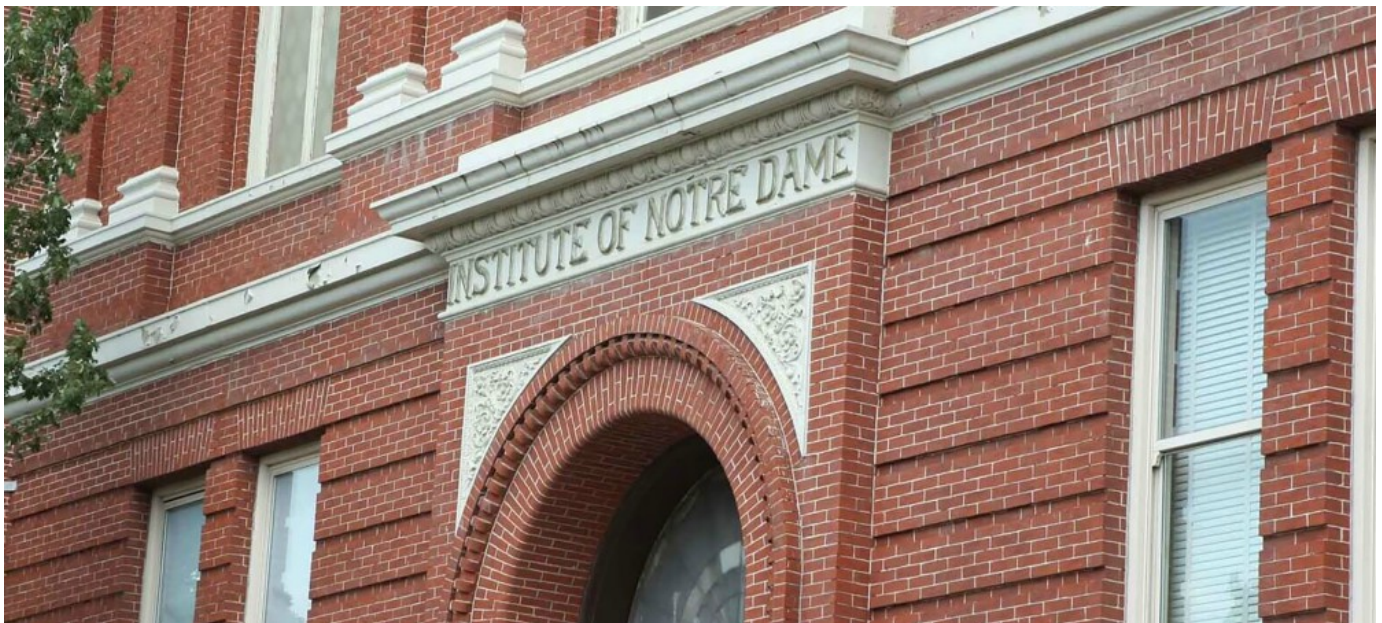
The exterior of the Institute of Notre Dame in Baltimore (CNS/Catholic Review)
