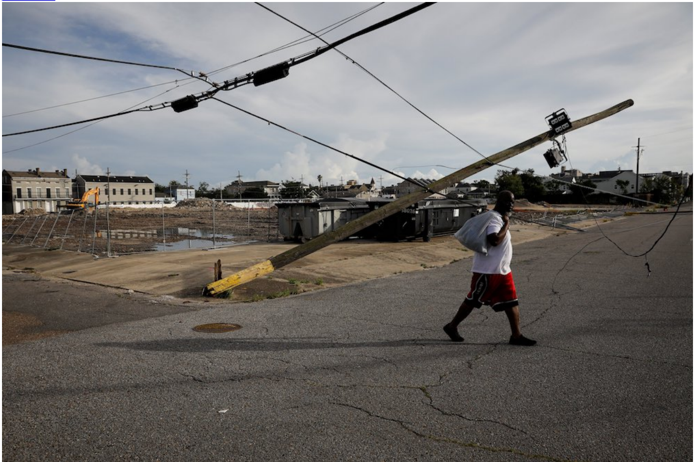
A man in New Orleans walks past a damaged electric line Aug. 30, after Hurricane Ida made landfall. (CNS photo/Marco Bello, Reuters)
