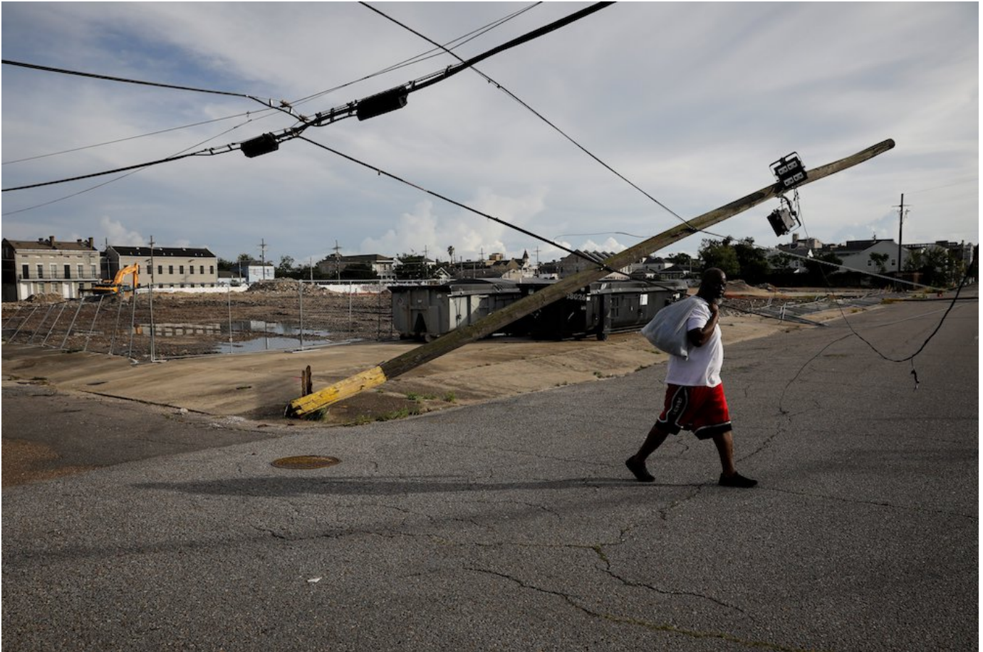
A man in New Orleans walks past a damaged electric line Aug. 30, after Hurricane Ida made landfall. (CNS photo/Marco Bello, Reuters)
