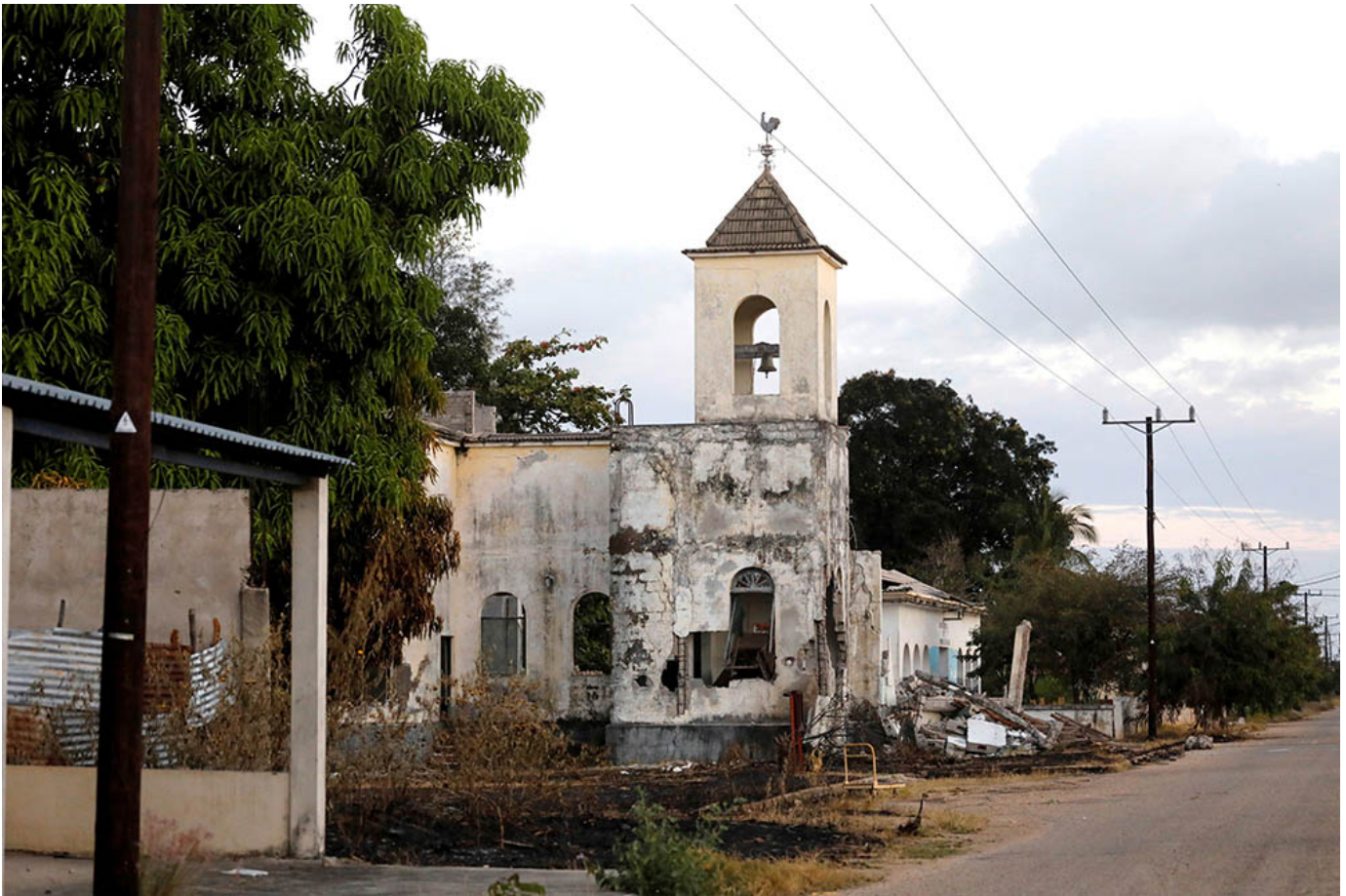
A church damaged by fighting is seen in Mocímboa da Praia, Mozambique, Sept. 22, 2021. (CNS/Reuters/Baz Ratner)
