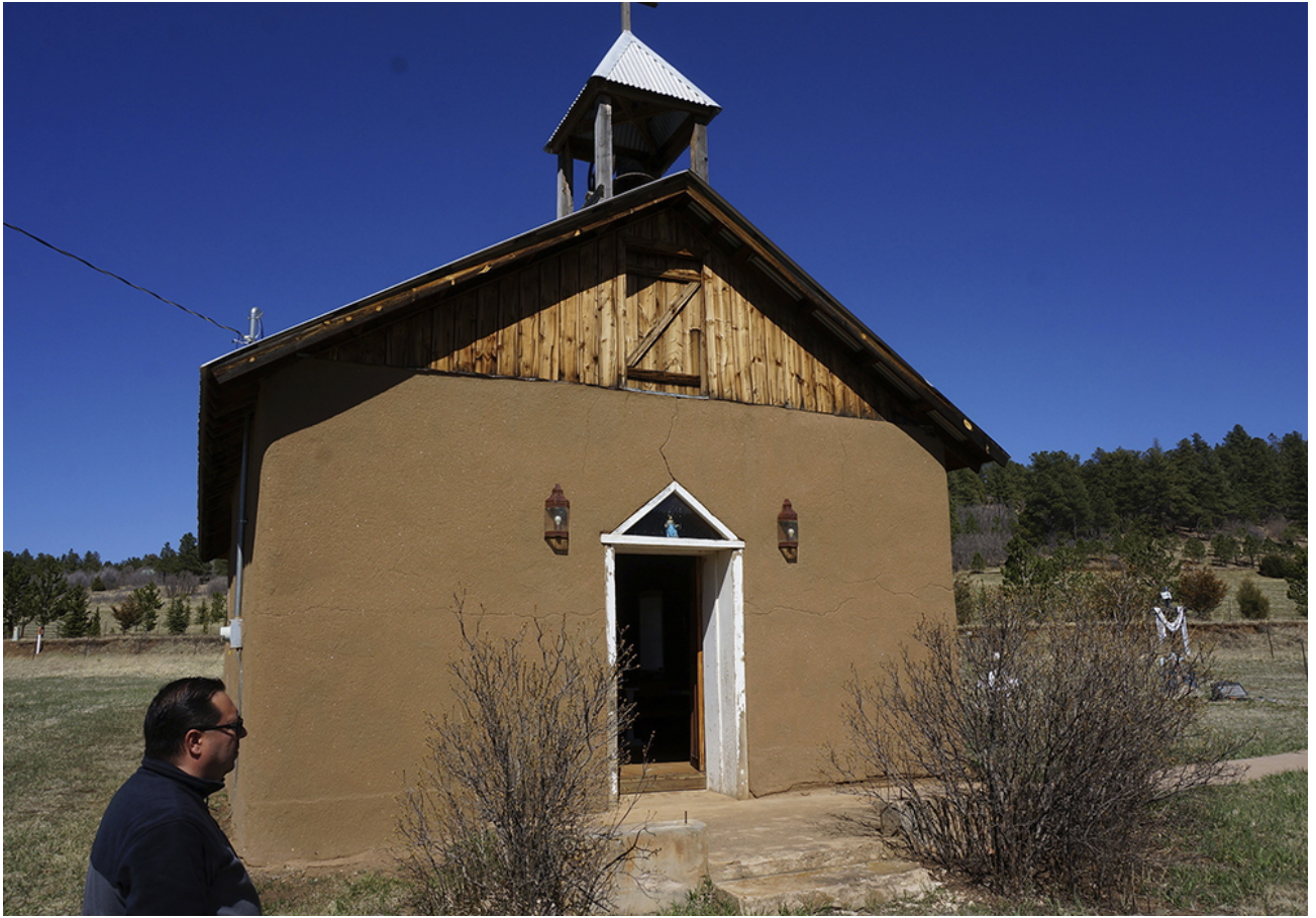
Fidel Trujillo stands outside the Santo Nino de Atocha Church in the remote mountain hamlet of Monte Aplanado, New Mexico, April 15. Trujillo serves as "mayordomo" or caretaker for a nearby church, also made in adobe — the sand, dirt and straw mix with which Catholic churches have been built here since the area was a remote outpost of the Spanish empire four centuries ago. (AP Photo/Giovanna Dell'Orto)
