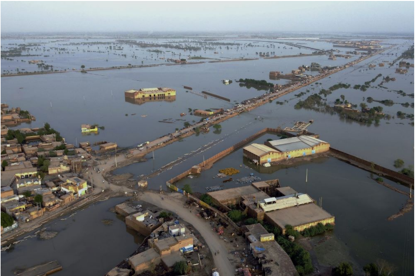
Floodwaters surround homes in Sohbat Pur city, a district of Pakistan's southwestern Baluchistan province, Aug. 29, 2022. (AP/Zahid Hussain)
