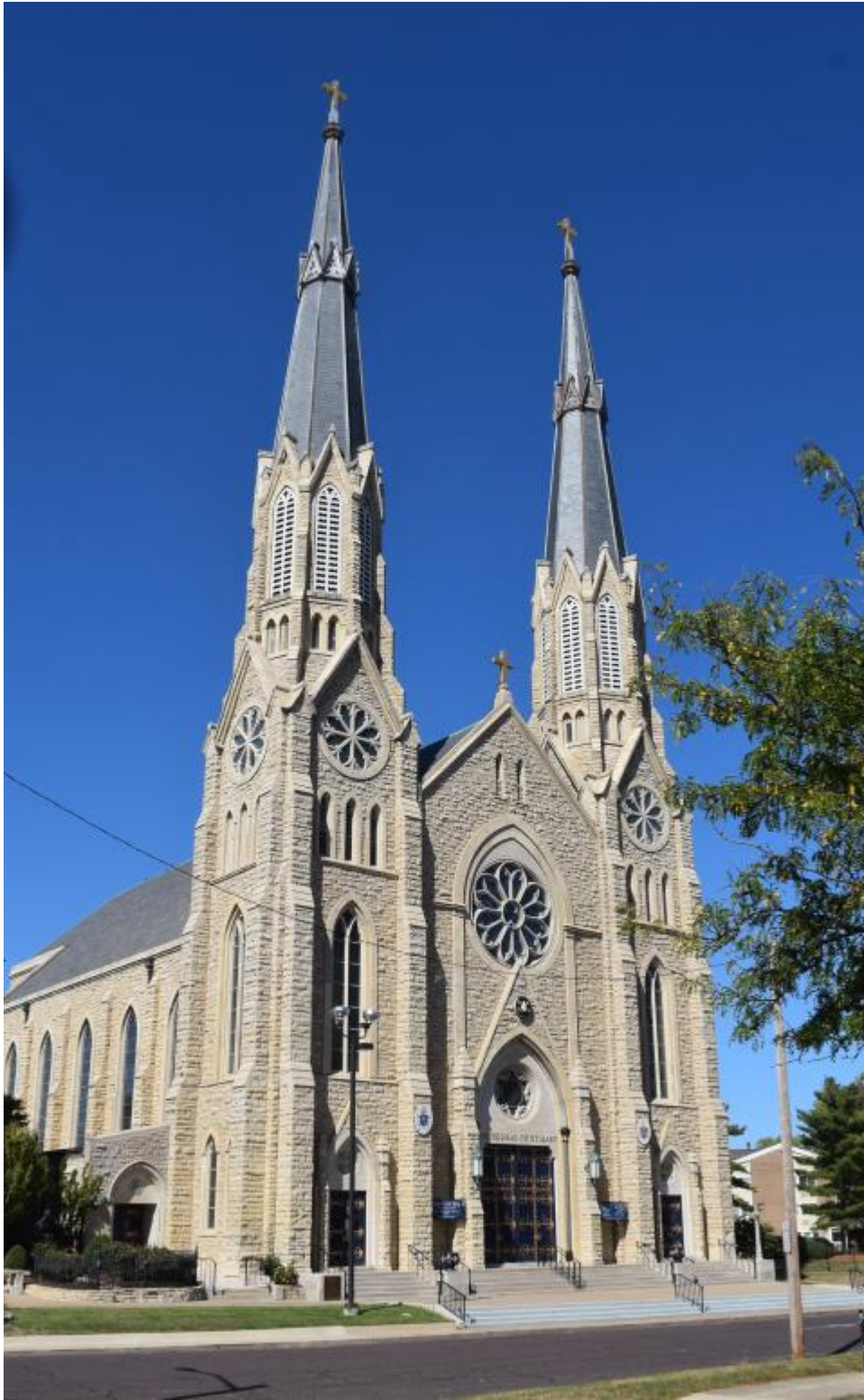
The facade of St. Mary's Cathedral in Peoria, Ill., is seen Sept. 28, 2017. The Diocese of Peoria announced May 18, 2024, massive restructuring plans that would merge its existing 156 parishes into 75 parishes with 129 "worship sites." (OSV News/Tom Dermody, The Catholic Post)
