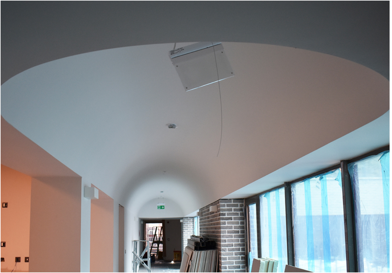
Vaulted ceilings along the corridors of Kylemore's new monastery challenged the plasterers creating the interior spaces. (Julie A. Ferraro)
