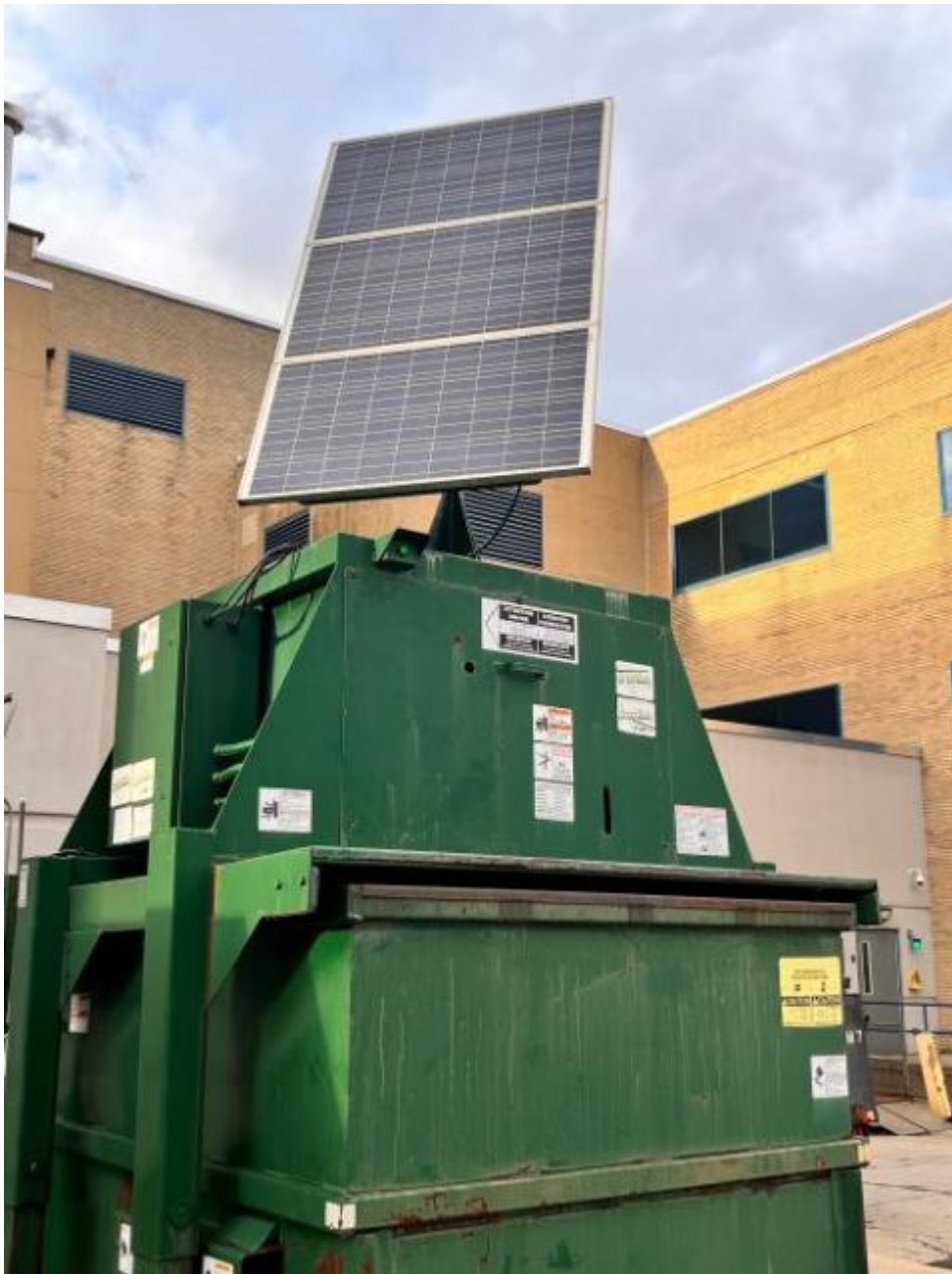
Solar power fuels a waste disposal system at Canisius University (George Cassidy Payne)
