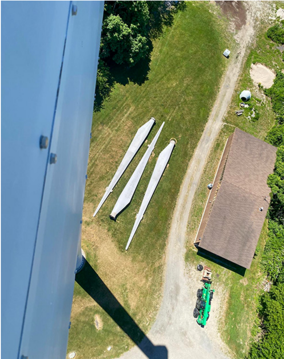
The blades for Portsmouth Abbey's wind turbine lie on the ground in 2026, waiting for repair after 20 years of function. (Courtesy of Joseph Byron)
